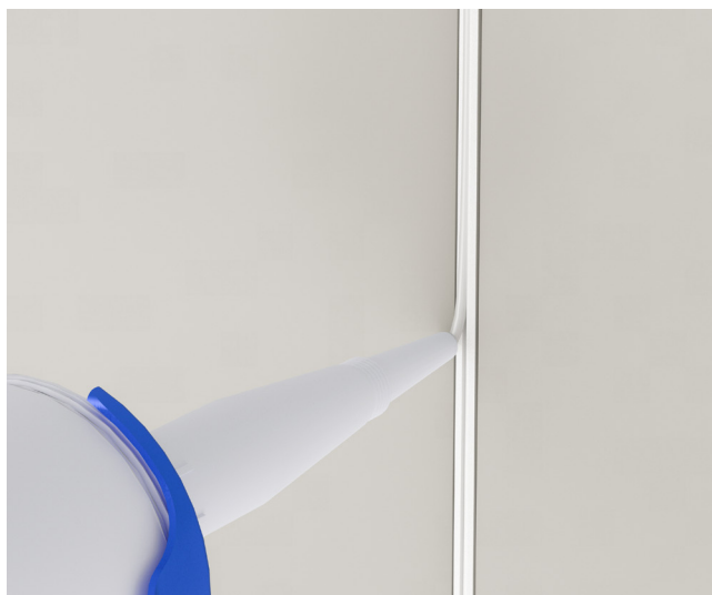
Seal the gap between the frame and the tiles.
